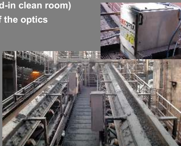
blast furnace equipped with Mineral LIBS
